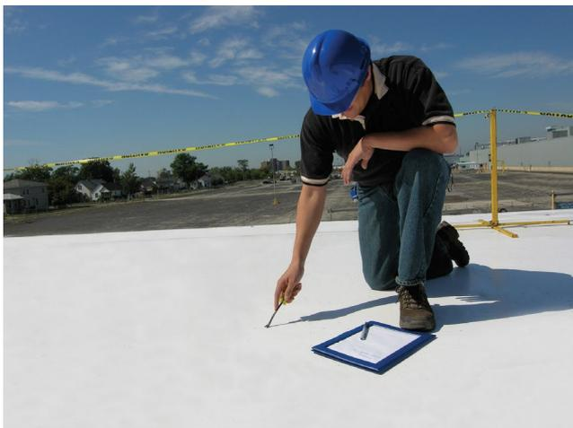
Duro-Last’s factory controlled custom prefabrication eliminates up to 85% of field seams, resulting in lower on-site labor costs and easier installation.
